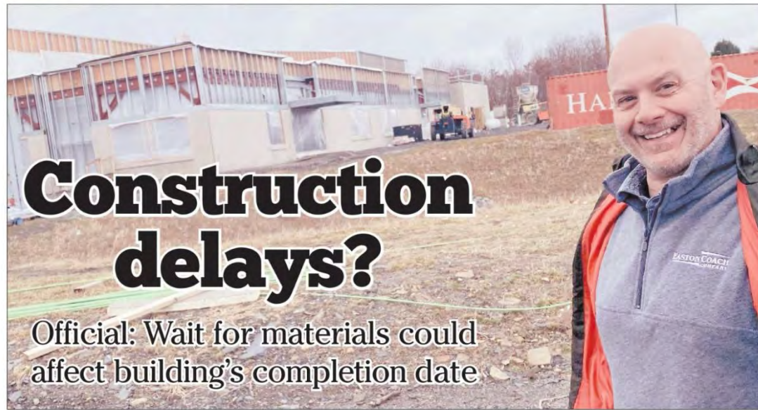
HAZLETON PUBLIC TRANSIT BUS FACILITY
